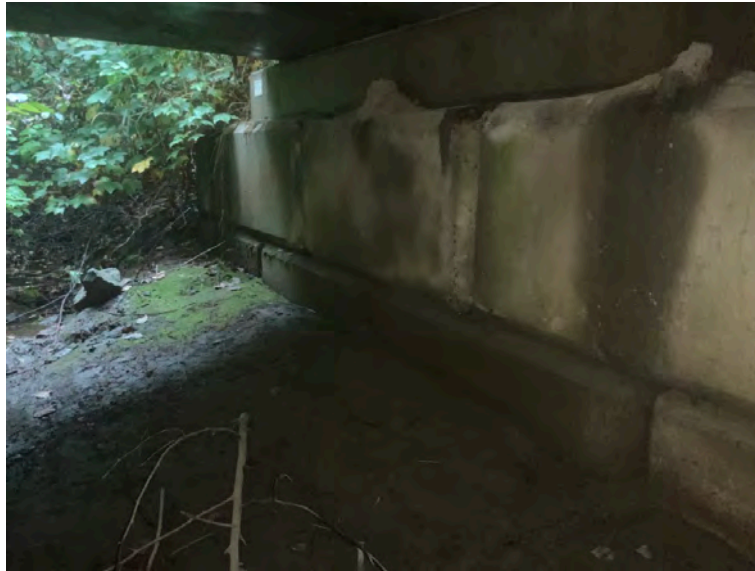
Left Bank Abutment when facing downstream
