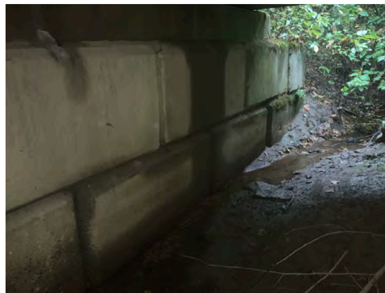
Right Bank Abutment when facing downstream
