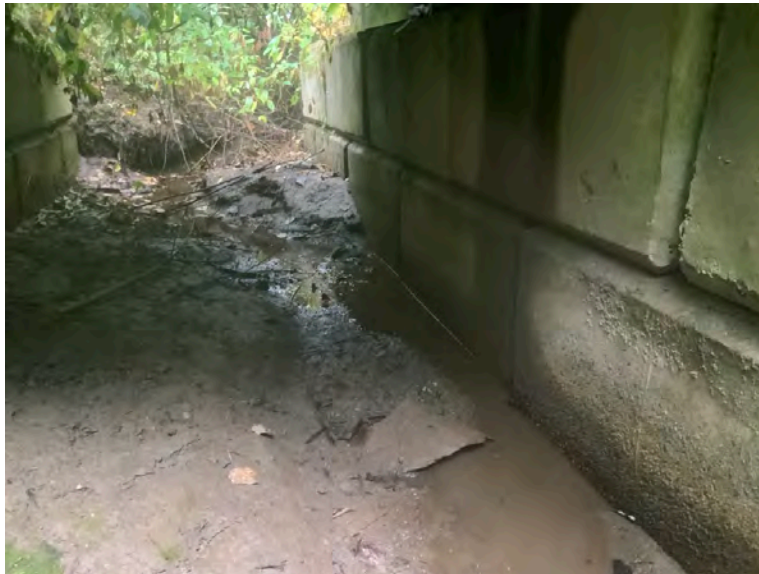
Right Bank Abutment when facing downstream
